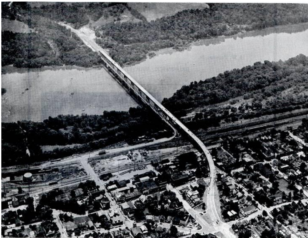
Figure 44. The new concrete bridge built in 1955 situated next to the old bridge before the city razed it. Courtesy of the Frederick County Archives and Research Center.
