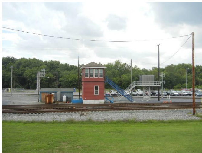
Figure 36. W.B. Tower as seen from Railroad View Park.
