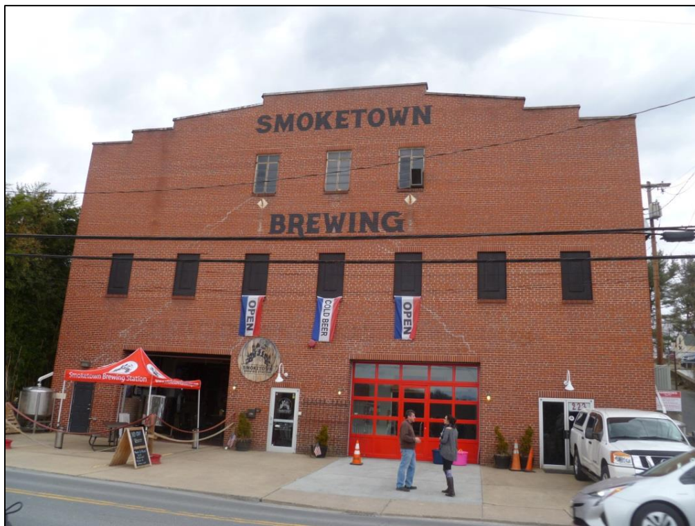
Smoketown Brewing Station (in old fire station)
